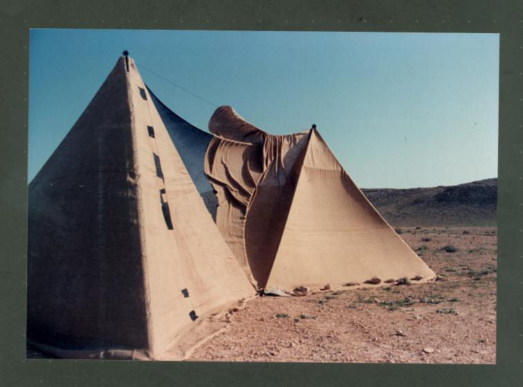
The doubled envelope is made of nylon mesh and burlap, creating variable patterns of transparency, light and shade. The black mesh inside soothes the eyes against the daytime glare.
